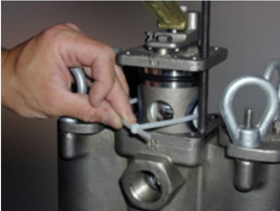
Photo 5: The first restraining tie is put into place to hold the ball, seats and seals in place before clearing the strainer body.
